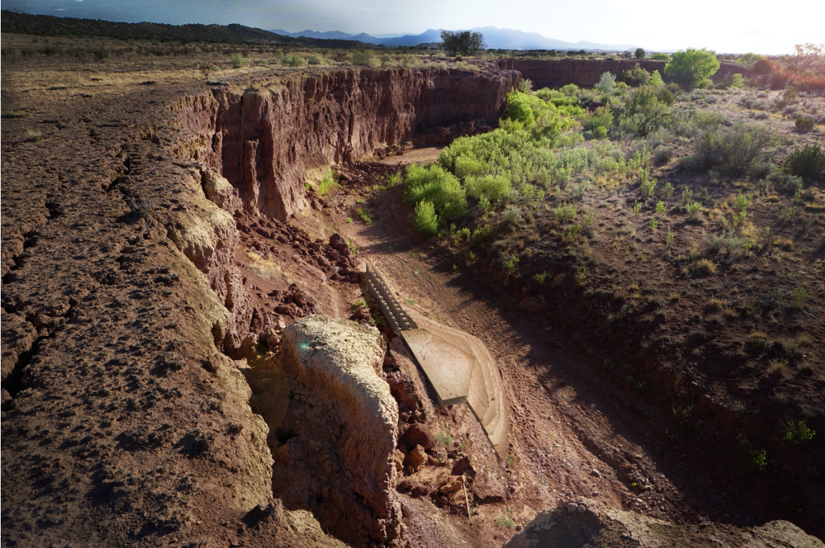
Figure 8: Conceptual rendering of third deflector with post baffle (Image by Ryan Bromberg)
