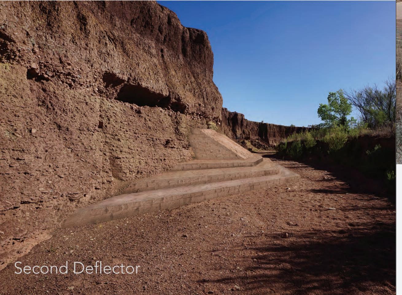
These are conceptual renderings of three different iterations of a functional deflector that pushes streamflow towards the opposite bank. The deflectors work to reintroduce meanders to the stream channel, which slow the flow of water, reduce streambank erosion, and reconnect the stream to a flood plain that provides riparian habitat for wildlife.
