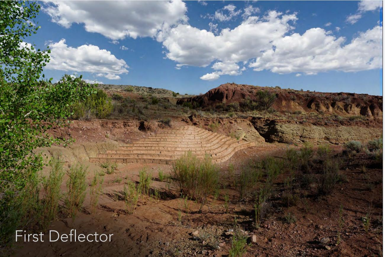
The stepped form allows the deflectors to function at various stream depths. The posts allow sediments and other materials flowing downstream to collect and fortify the stream bank.
