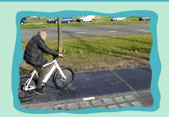
Solar paving modules will be installed on some parts of the bike path, throughout the Esplanade. This will not only provide power to light the road at night, but also raise awareness of renewable energy sytems.
