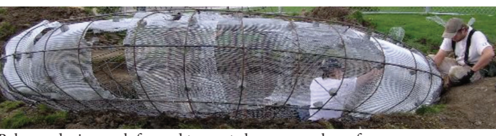
Rebar and wire mesh formed to create large amorphous forms
