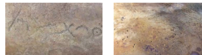
Concrete shell allows for detailed finishing techniques
