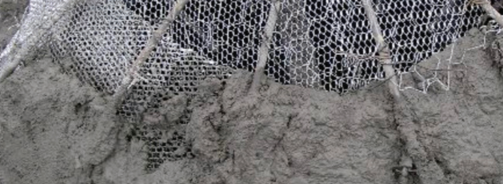
Rebar and wire mesh coated with concrete to create final form
