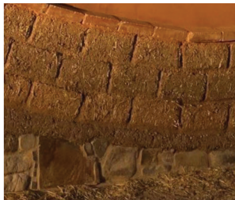
Stone and sunfired clay brick inspiration for materiality of sections of the serpentine form
