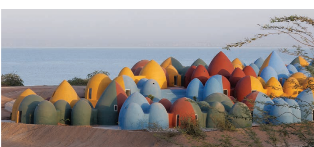
Inspiration for domed forms. Hormuz, Iran. ZAV Architects employed the adobe techniques of master Nader Khalili (1936-2008).
