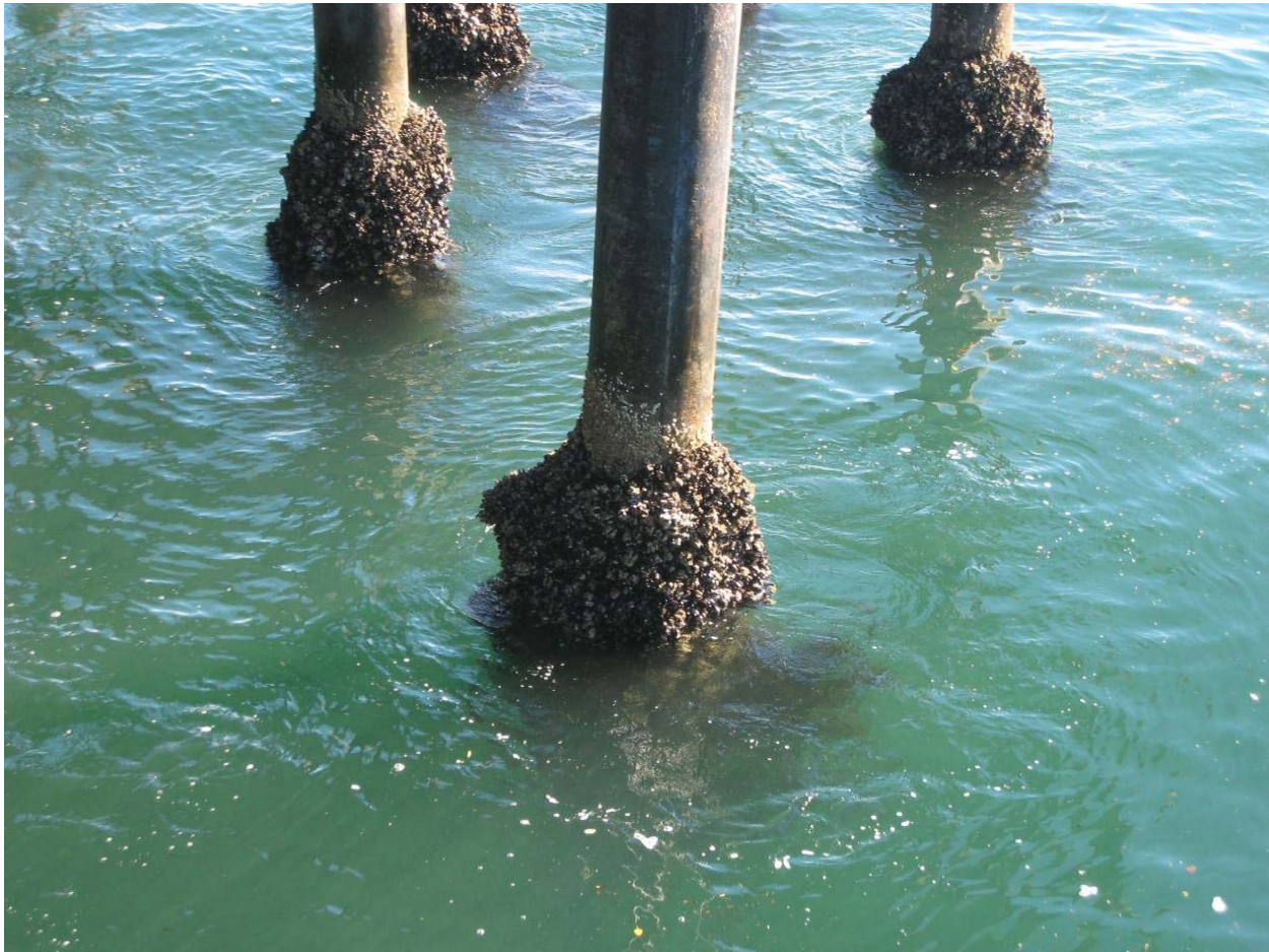
Figure 10. Barnacle and Mussel Community on Pilings.
