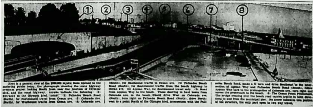
Newly constructed Viaduct and associated transportation infrastructure, Colorado Grade Separation Project (Santa Monica Evening Outlook, "Opening of Overpass Marks Completion of Half Million Dollar Highway Link," June 27, 1940, p. 1.)
