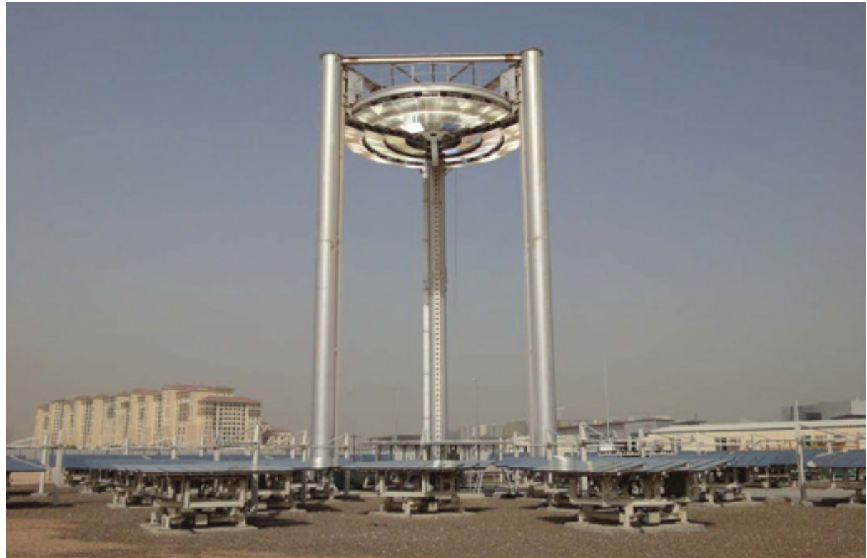
Beam-down point-focus CSP heliostat array at Masdar
