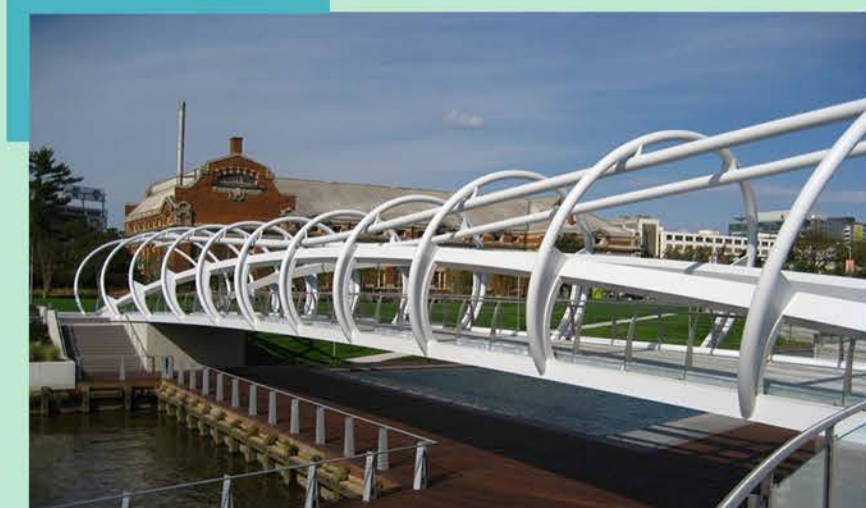
PEDESTRIAN BRIDGE OVER THE JACKA BOULEVARD
