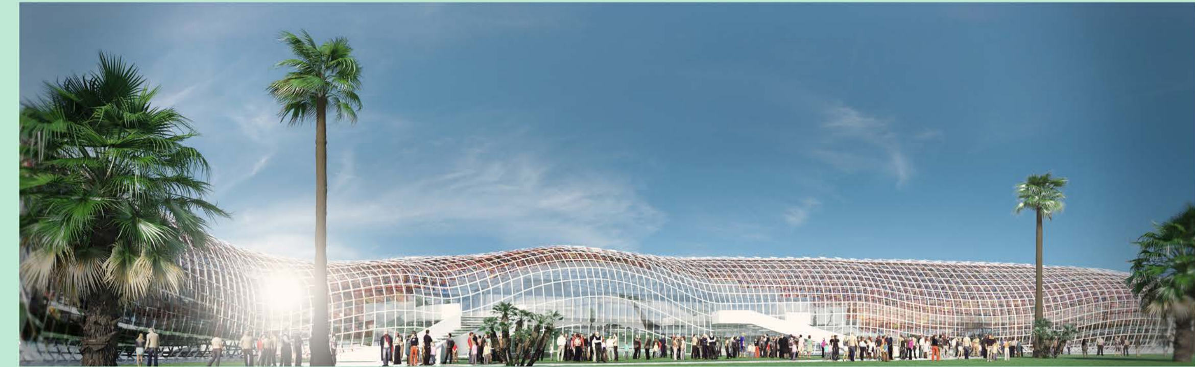
NORTH FACADE WITH COLORED, ENERGY GENERATING SOLAR PANELS
